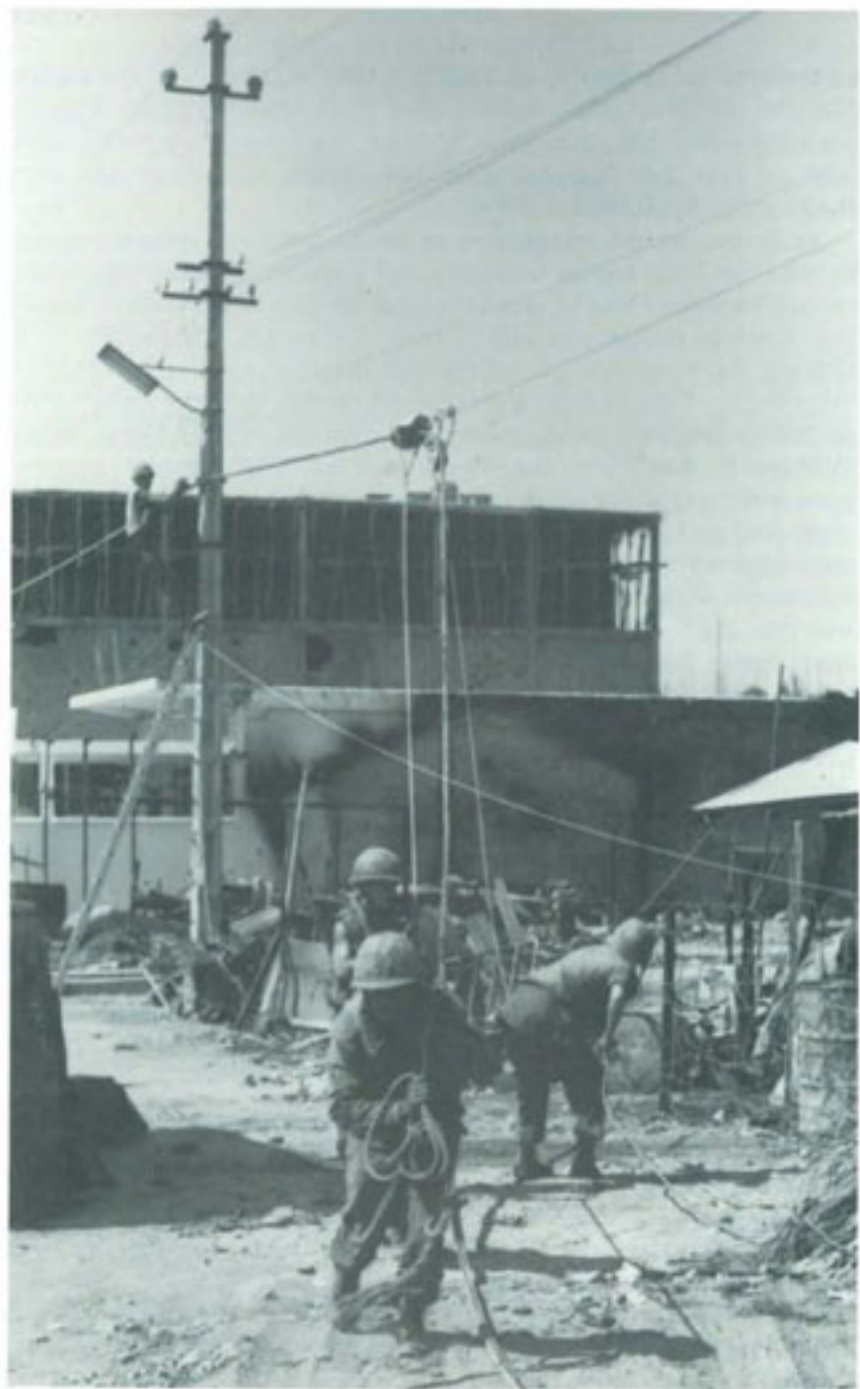
CABLE TEAM AT WORK DURING TET OFFENSIVE
