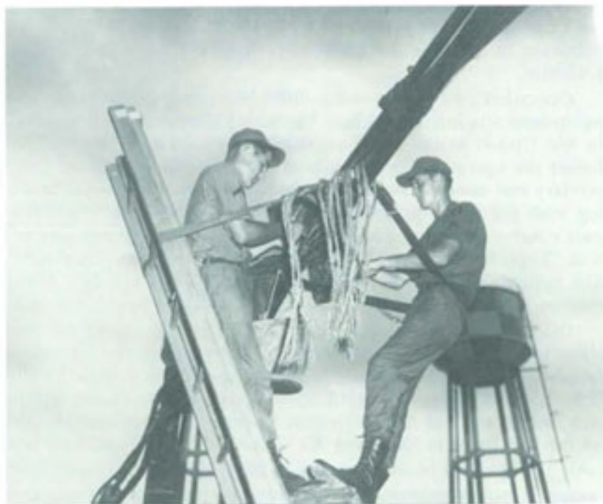
CABLE-SPLICERS AT WORK AT A LARGE FIXED BASE
