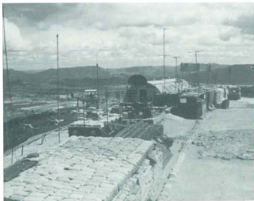
HON CONG MOUNTAIN SIGNAL SITE, focal point for integration of 1st Cavalry Division communications and 1st Signal Brigade's Corps Area Communications System.
