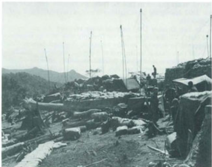
FIRE SUPPORT BASE ON A RIDGE NEAR DAK TO. Tall antennas were used to extend range of mobile voice radios.
