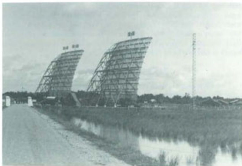
BILLBOARD ANTENNAS OF THE BACK PORCH SYSTEM AT PHU LAM IN 1962. On top of the 60-foot tropospheric scatter antennas are the smaller antennas for mobile combat equipment that provided the "tails," or extensions.
