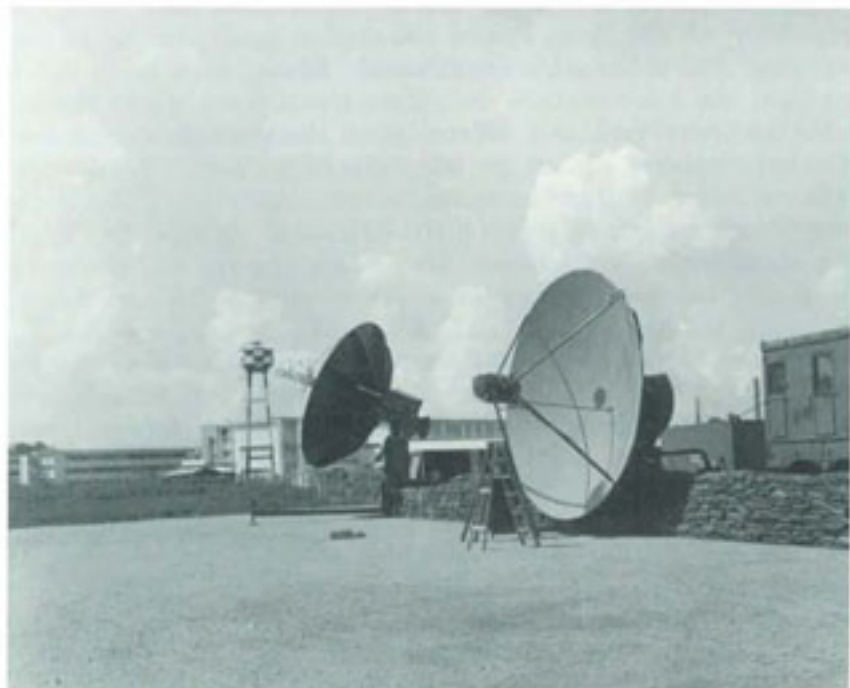
FIRST SATELLITE TERMINAL, BA QUEO, NEAR SAIGON. This station linked Vietnam with Hawaii in first use of satellite communications in a combat zone.
