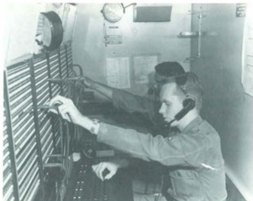
SIGNALMEN OPERATING MOBILE MANUAL SWITCHBOARD IN 1962
