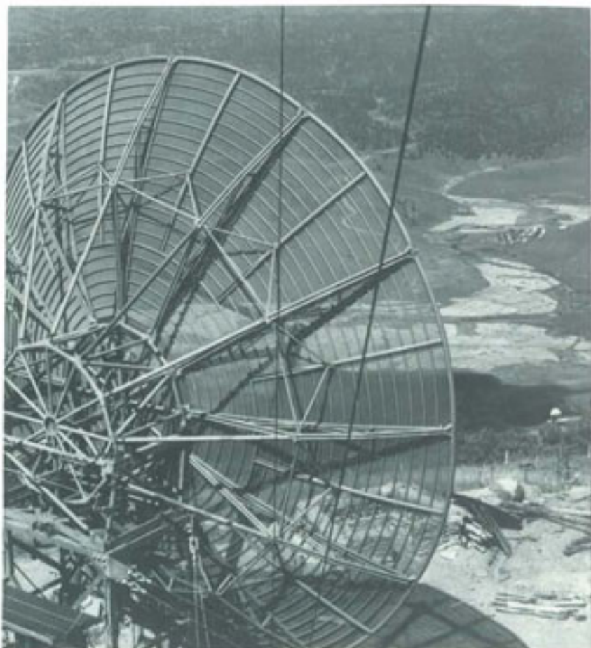
MOBILE TROPOSPHERIC SCATTER ANTENNA ON NUI LANG BIAN NEAR DALAT was installed and defended by U.S. Army Signalmen in late 1965.
